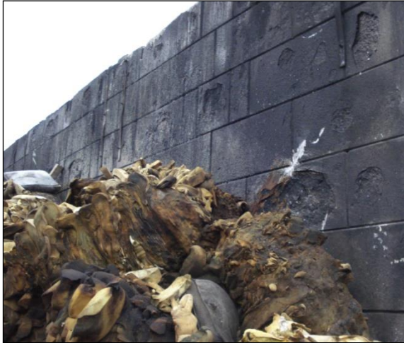
Illustration 4: spalling damage
